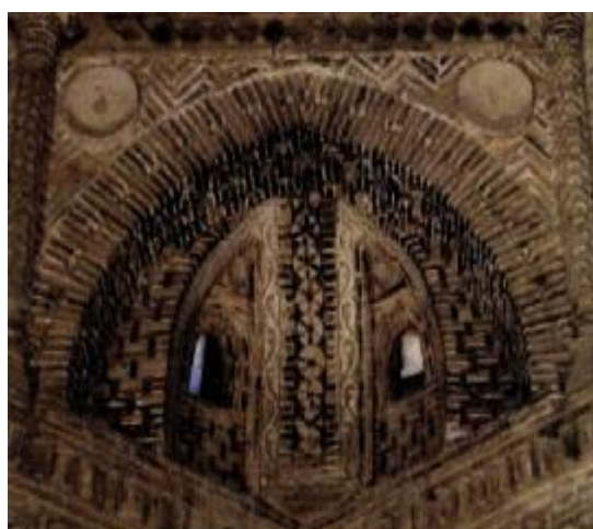
Fig. 6 Interior view, squinch supporting the dome (Ibid)
