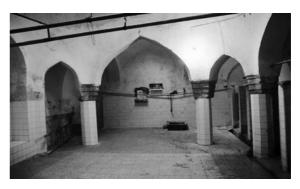
Picture 5 Small hot-house, Haj kazem bath - In Qajar period, the change of the function of water reservoir made the dimensions of the hot-houses smaller.(Photograph by author)
