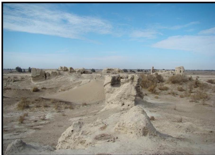
Figure 10. Zahedan-e Kohneh: tower in the northeast corner of the castle (by the authors).
