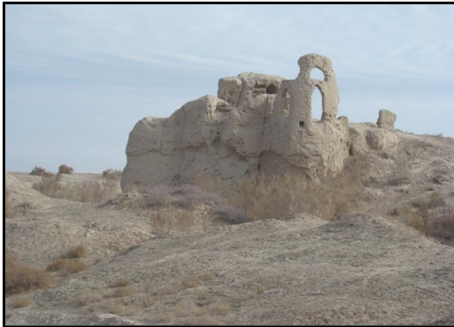
Figure 7. Zahedan-e Kohneh: tower in the northwest corner of the castle (by the authors).
