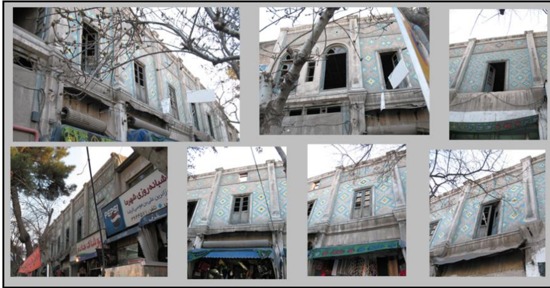
Fig. 5A. Real pictures of Astan-e Quds house facade
