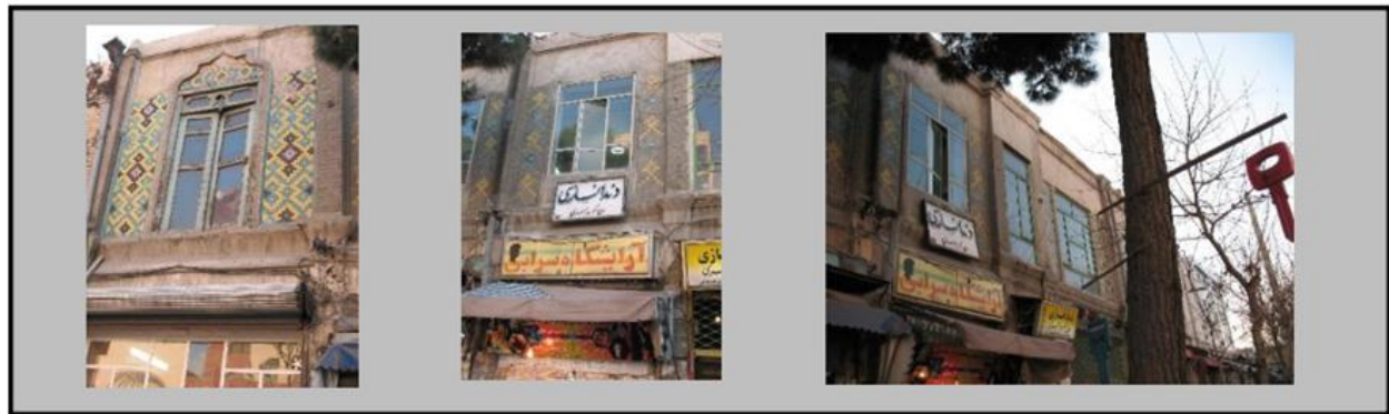
Fig. 6A. Real picture of Javaheri house façade
