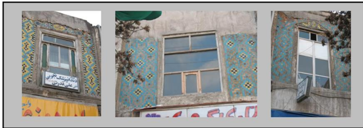
Fig. 9A. Real pictures of Shahr-dari house façade
