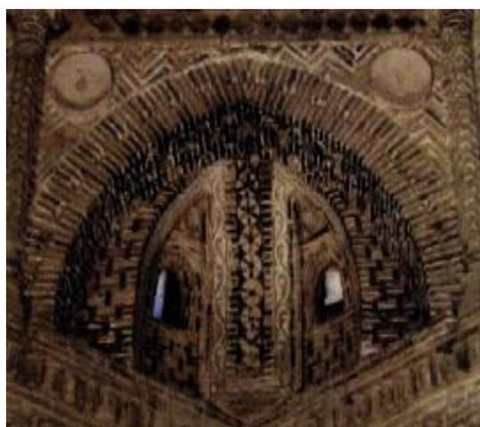
**Fig. 6** Interior view, squinch supporting the dome (Ibid)
