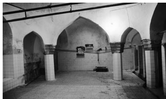
Picture 5 Small hot-house, Haj kazem bath – In Qajar period, the change of the function of water reservoir made the dimensions of the hot-houses smaller. (Photograph by author)
