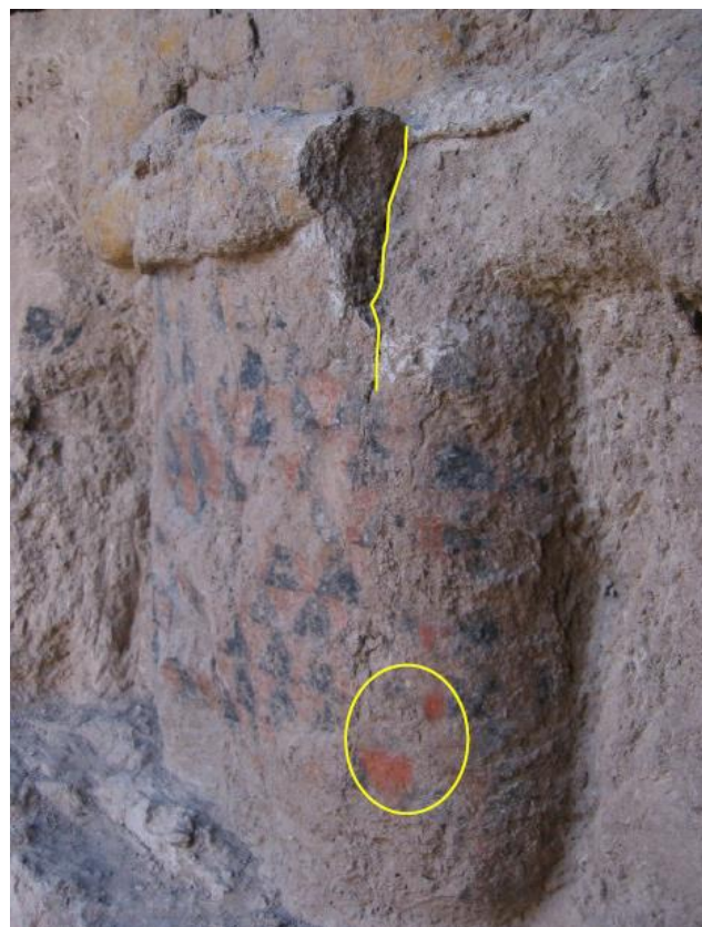
Fig. 10. Fall of left forearm of the relief and continuous crack in hand-wall interface (Author, 2006).
